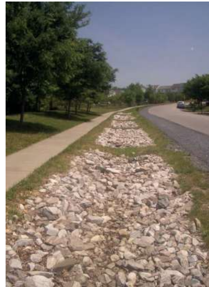
Fig.2. Stone infiltration trench in the city
